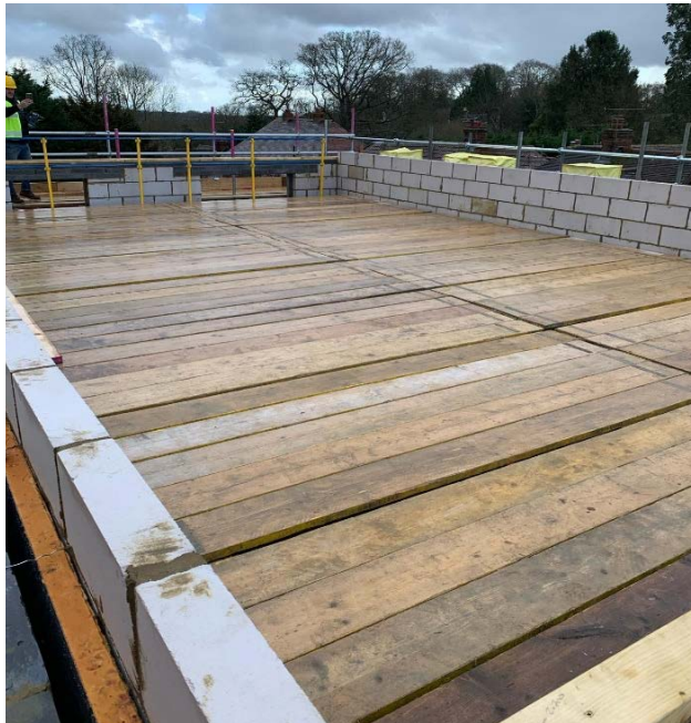
Roof Trusses (Decking at platform height 1.8m)
