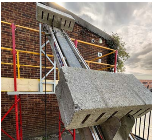
Loading out by Hoddi/ Bumpa Hoist
