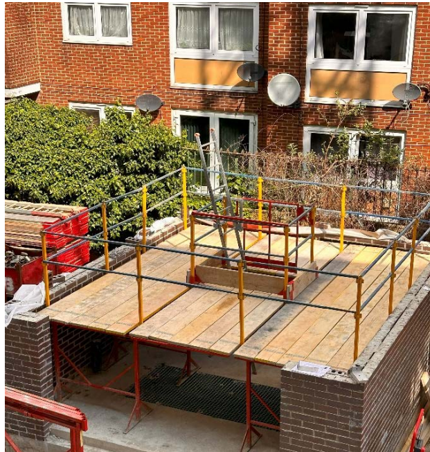
Sub-Station (Decking at platform height 1.7m)
