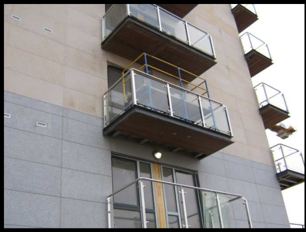
Balcony Soffit Cladding (John Fleming Construction, Dublin)
