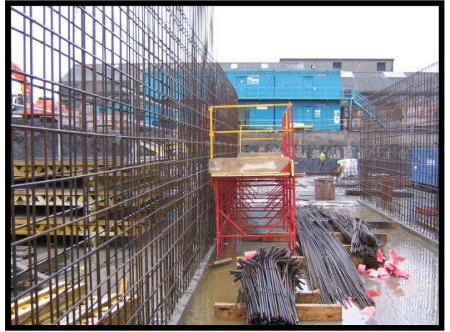
Steel fixing (Daninger Construction Ltd)
