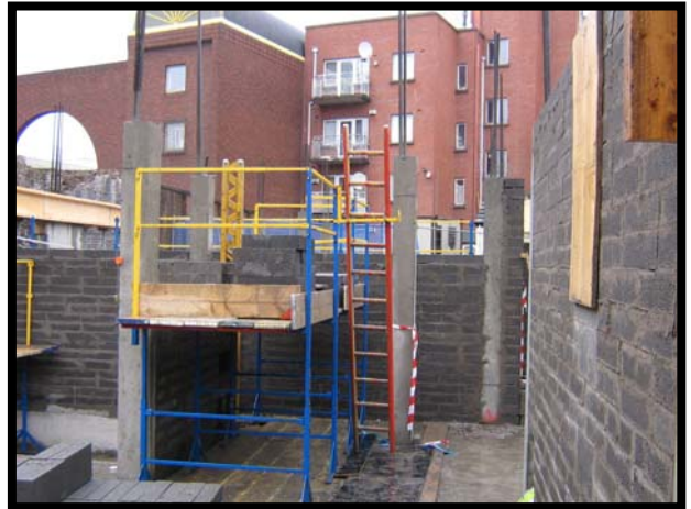
Blocklaying (BAM Construction Ltd)
